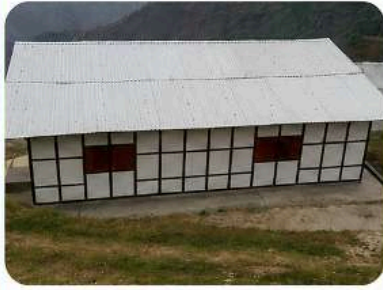
Large Corrugated Shed
