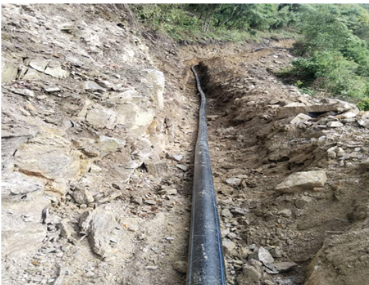
Trench laying of HDPE, Gayrikha scheme in Haa PemaGatshel
