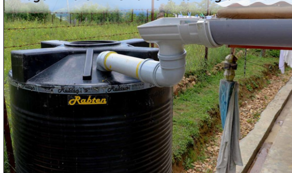
Figure 6: Roof rainwater harvesting system for 10 households in a women's group in Chubjekha village in Paro. BF Small Grants Program
