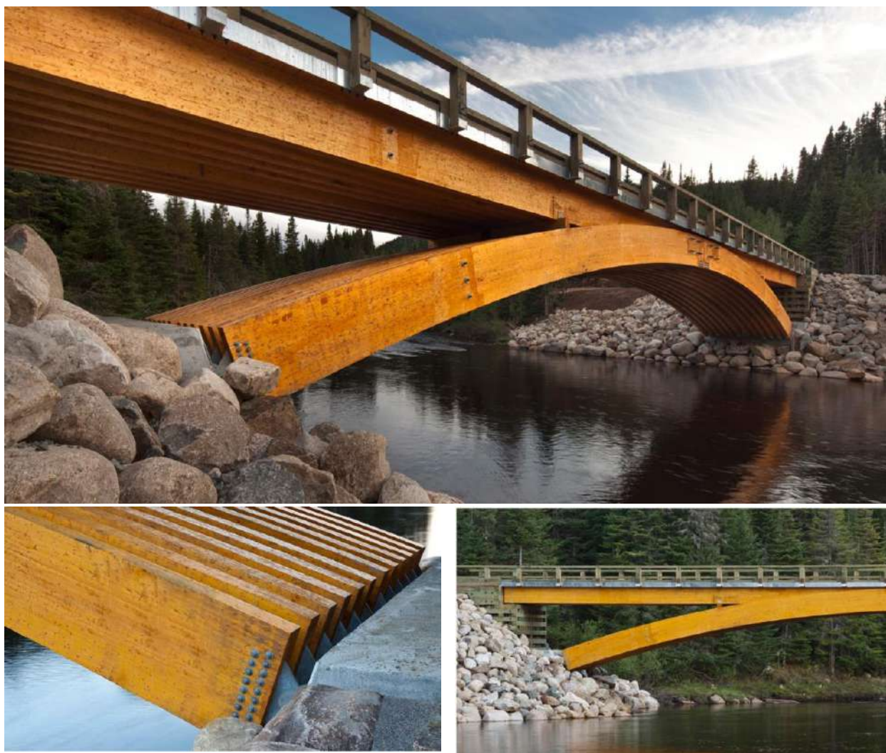
Plate 4. Mass timber bridge in Montmorency Forest, Québec 12
