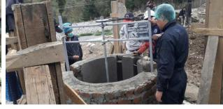
Figure 8: Construction of biogas plant
